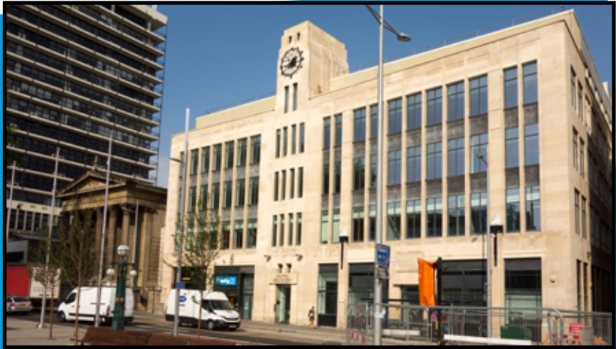
33 Colston House. (formerly Bristol Gas Company Showrooms) 1935, St Augustine's Parade.
