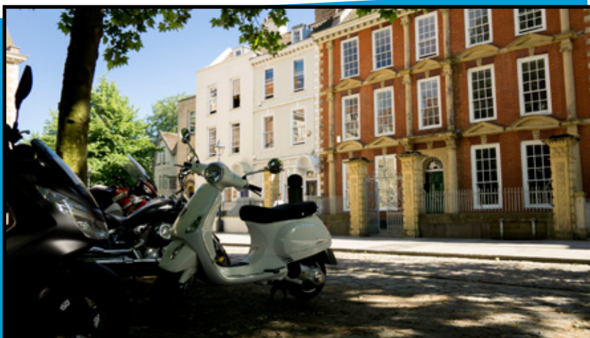
29 Queen Square, one of the few original properties remaining in its original state.
